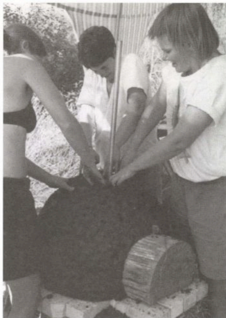
Pushing and "weaving" the cob into the previous layer.
