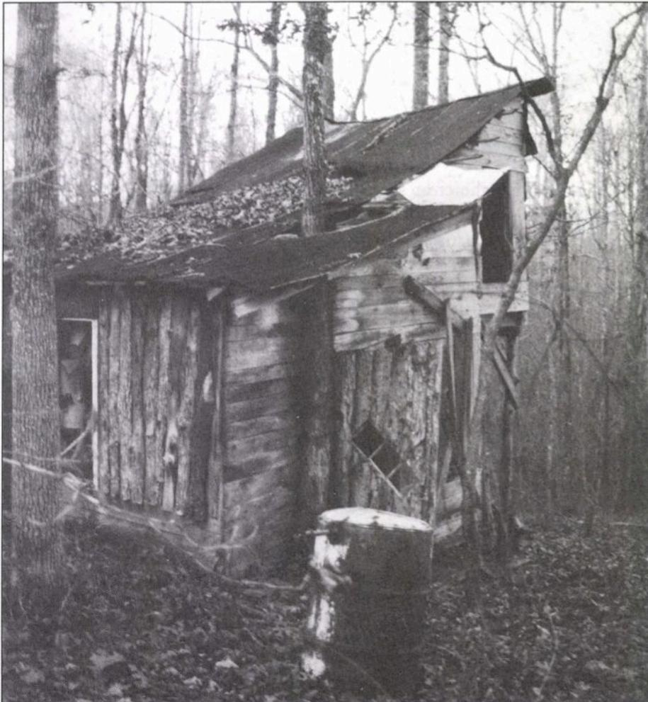
*A well-meaning communitarian built this inexpensive dwelling 20 years ago in Dunmire Hollow community, with a living tree growing through the roof, and diagonal, diamond-shaped windows in the door. With no foundation, the wood has rotted, and wind swaying the tree has gradually pulled the house apart.*
