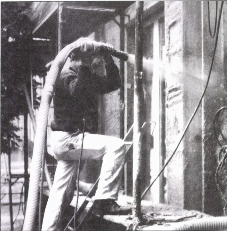
Niederkaufungen's construction company installs cellulose insulation, one of their specialties.
