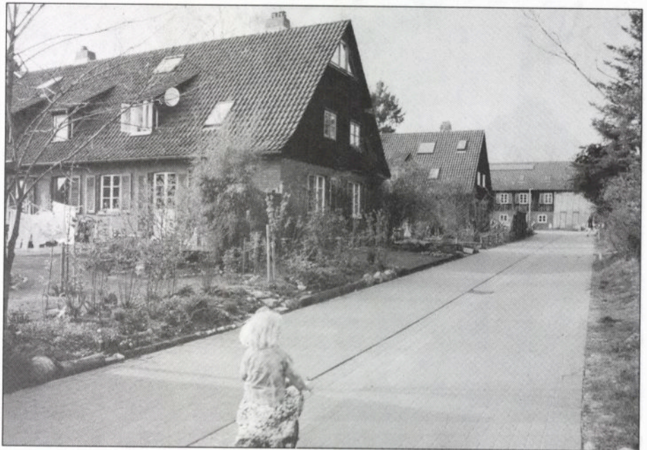
ABOVE: In this former factory housing complex the asphalt pavement has been torn up and replaced with brick. The center gutter uses less space for water runoff than paved shoulders.
