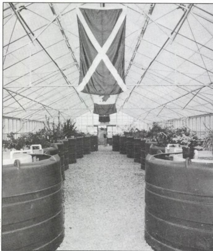
The “Living Machine,” (© Ocean Arks, International) a biological sewage treatment system at Findhorn.
