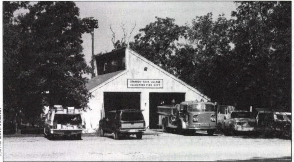
Members donated time, labor, skills, and money to build their community firehouse.
