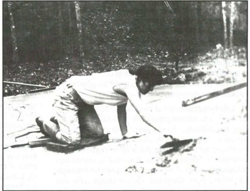
Donna working on a foundation at Twin Oaks.
