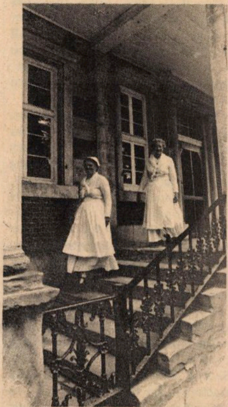
Number One House was made from sandstone quarried in the Society's own quarry, brick made from its own clay and iron railings made in its own furnace and foundry.
