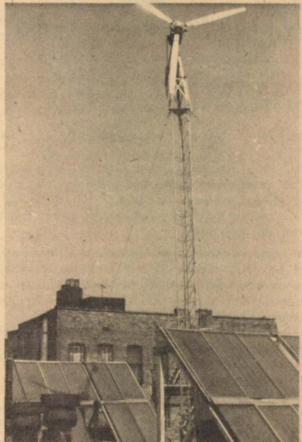
Windmill and solar collectors, 519 East 11th Street
