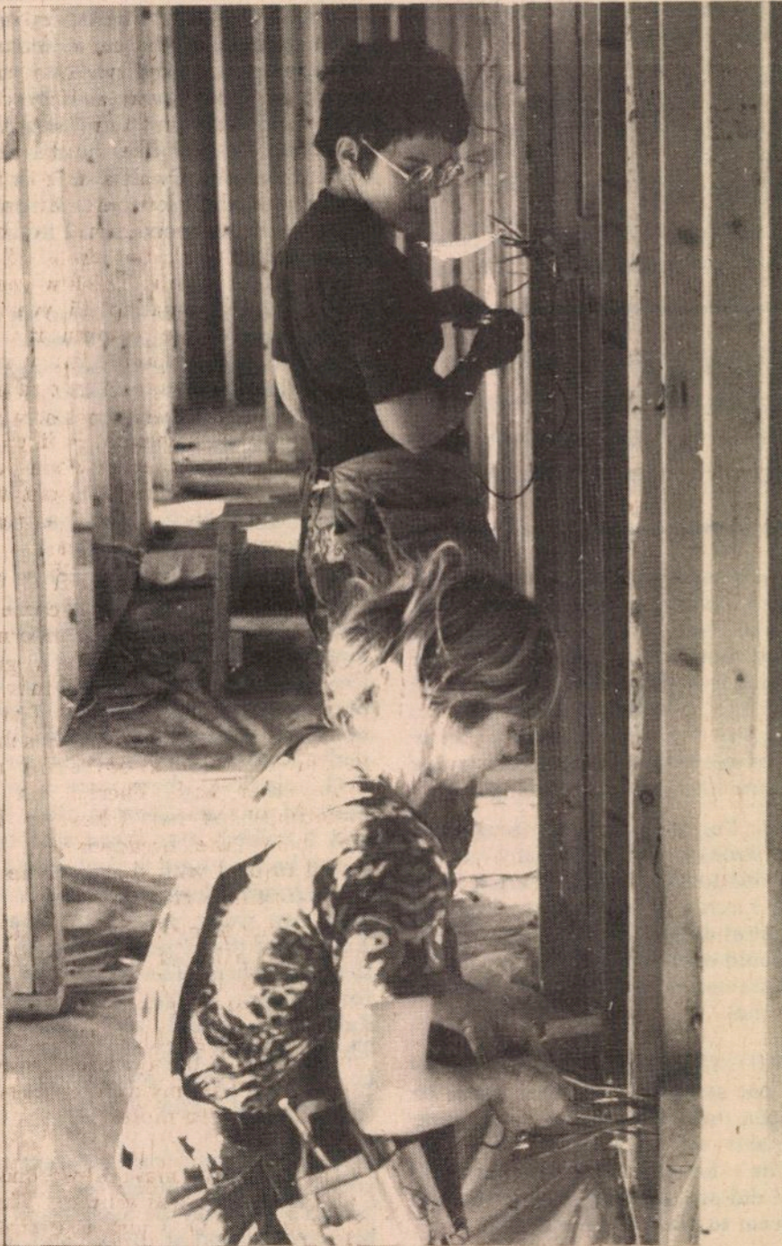
Bree and Linda on an electrical job
