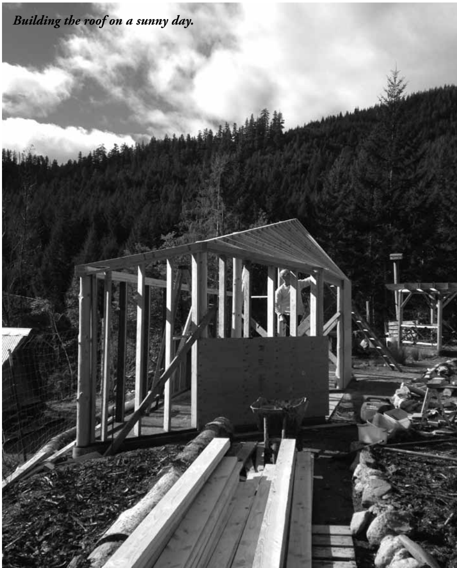
Greenhouse under construction overlooking one of the small cabins.
