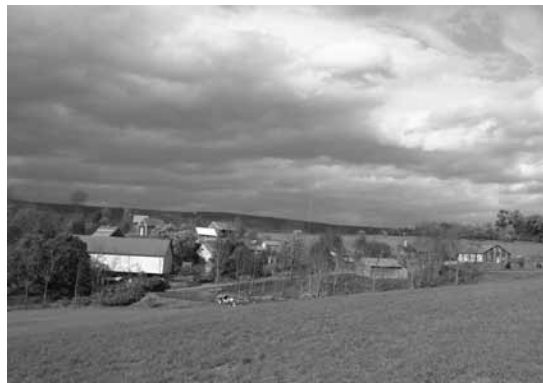
Left: The first four log buildings we constructed. Left to right, the Gemeinehaus, summer house, First House, and outhouse. Right: The Hermitage, with the master plan completed, as it appeared in 2011.
