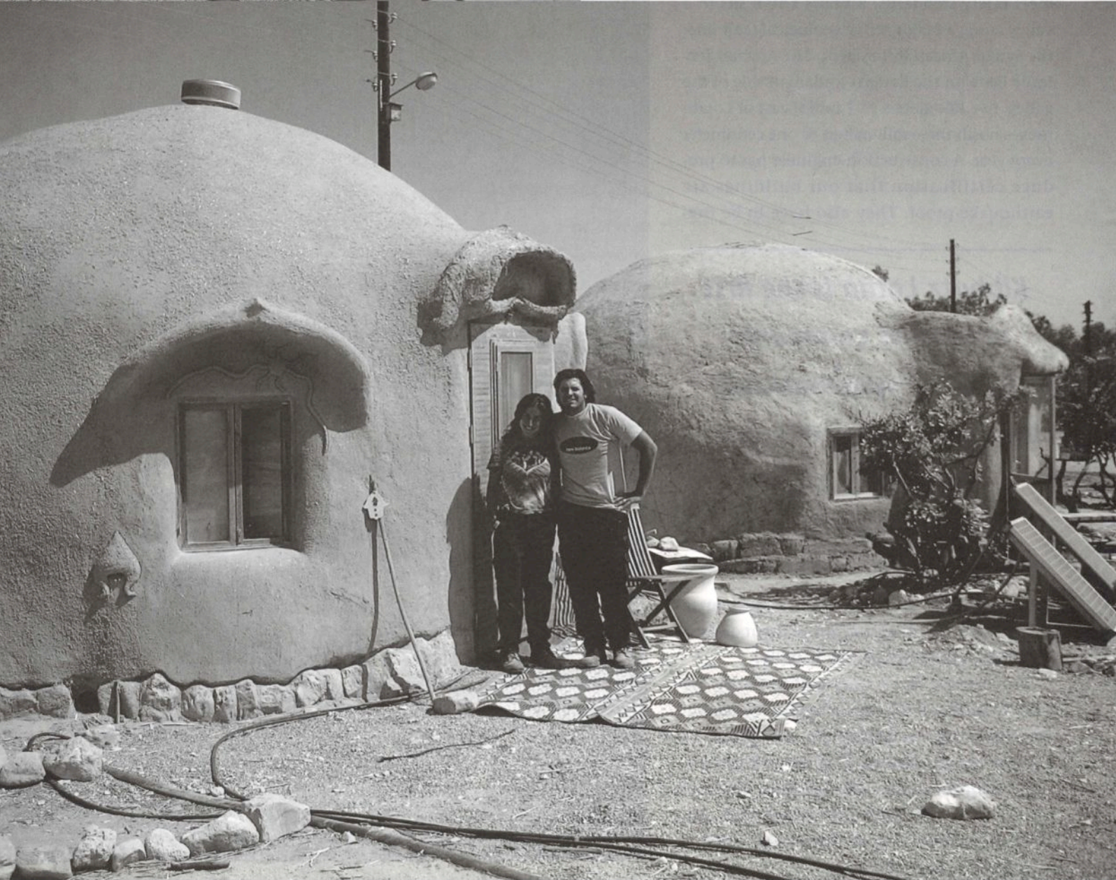
Top: Many lessons were learned during construction of the first three prototypes. The domes built in 2007, like the ones shown here, are hybrid geodesic domes with openings built in for windows and doors. The front extension will include shelves for storage. Bottom: Sheera and Ryan are Green Apprenticeship graduates who remained on Lotan to complete the dome that their group began to construct.
