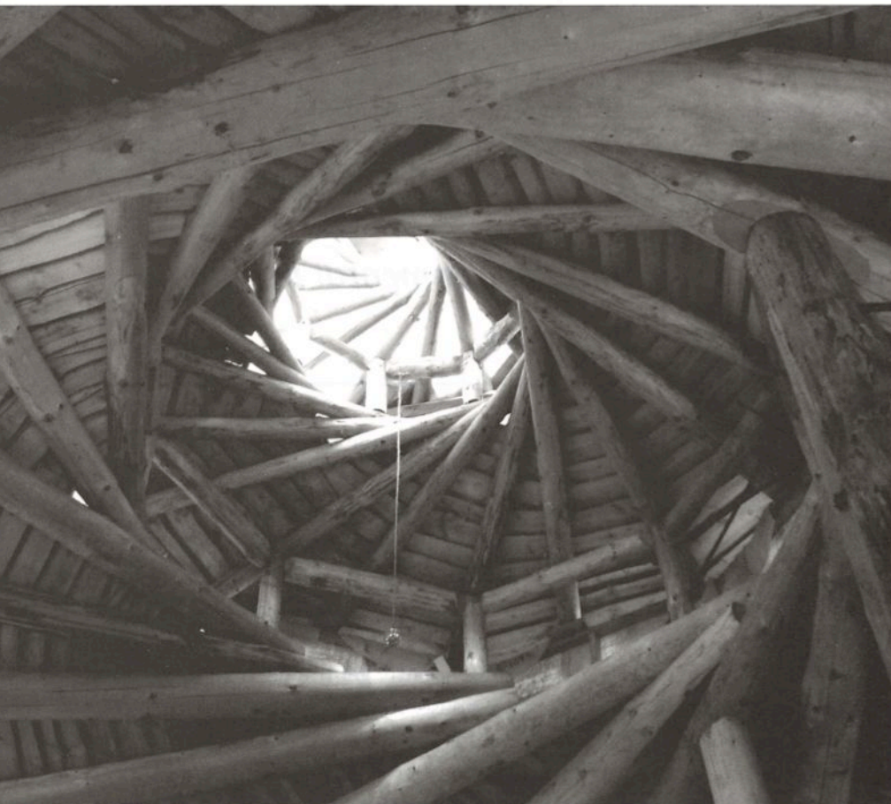
Top of the self-bearing beam construction on the Conch House, built by Morten and Hanne.
