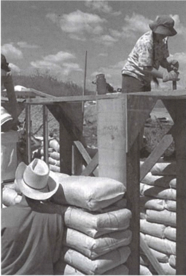
Community members built their new root cellar of earthbags for maximum earth-coupled mass.
