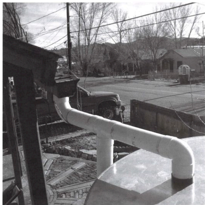
Andrew Millison catches water off his rooftop via PVC pipe from his raingutter to his front yard cistern.
