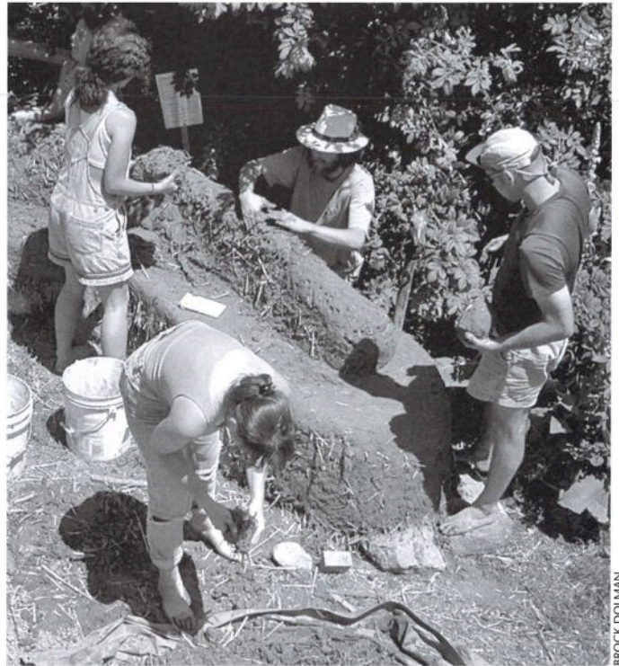
Participants of OAEC's school garden teacher training program learn to build a cob bench.
