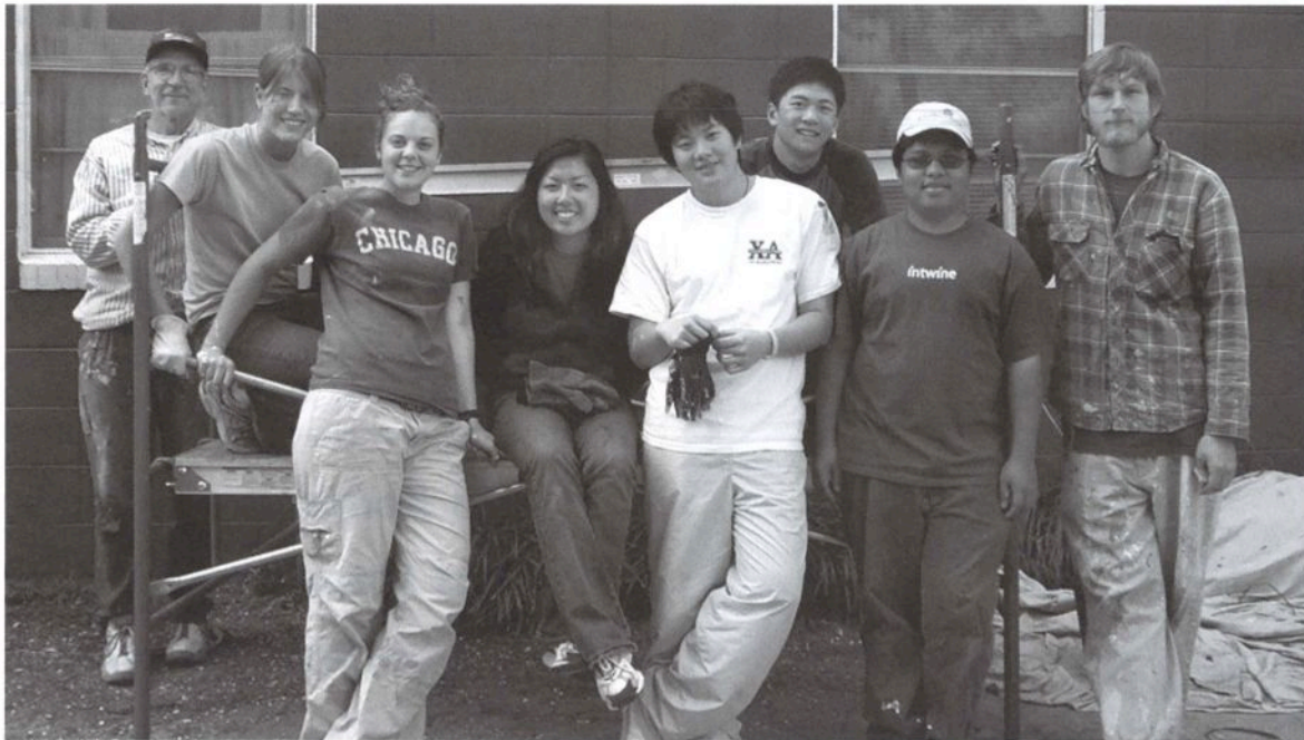
Taking a break from roofing and painting a neighbor's house, are (left to right) Koinonia member J. Reilly, "alternative spring break" students from the University of Virginia, and Arlen Daleske, a pastor on a service sabbatical at Koinonia.
