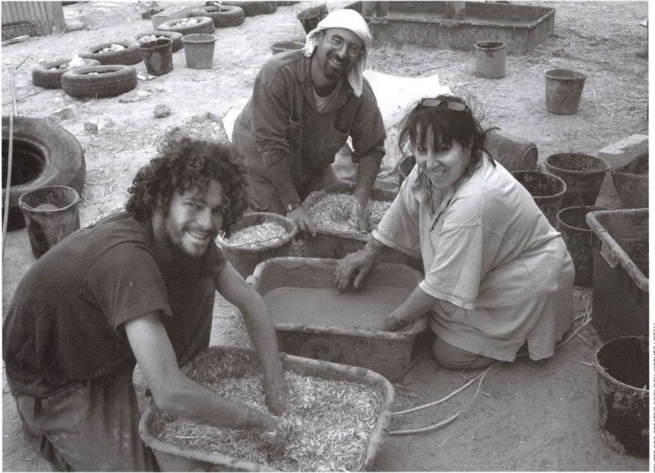
Mike (left) from Kibbutz Lotan, shows Bedouin villagers at Wadi el N'aam how to mix earthen plaster for the new clinic.
