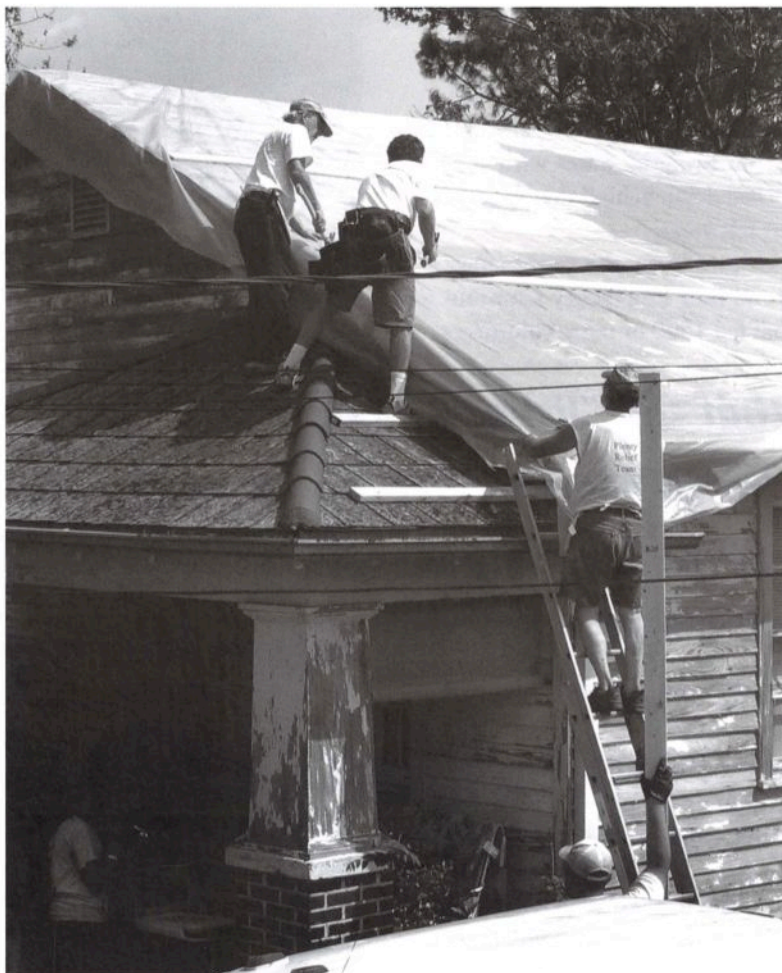
Plenty volunteers rain-proofed the roof of an elderly neighbor.
