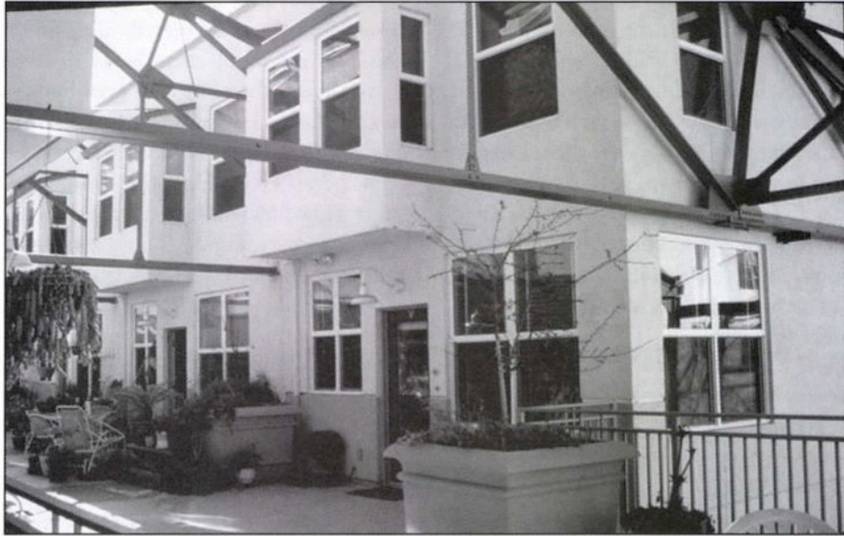
The original steel roof trusses were kept to conform to local regulations.
