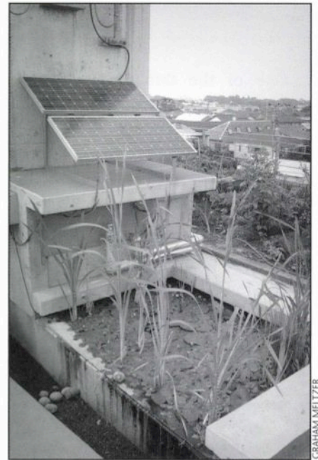
The constructed wetlands.
