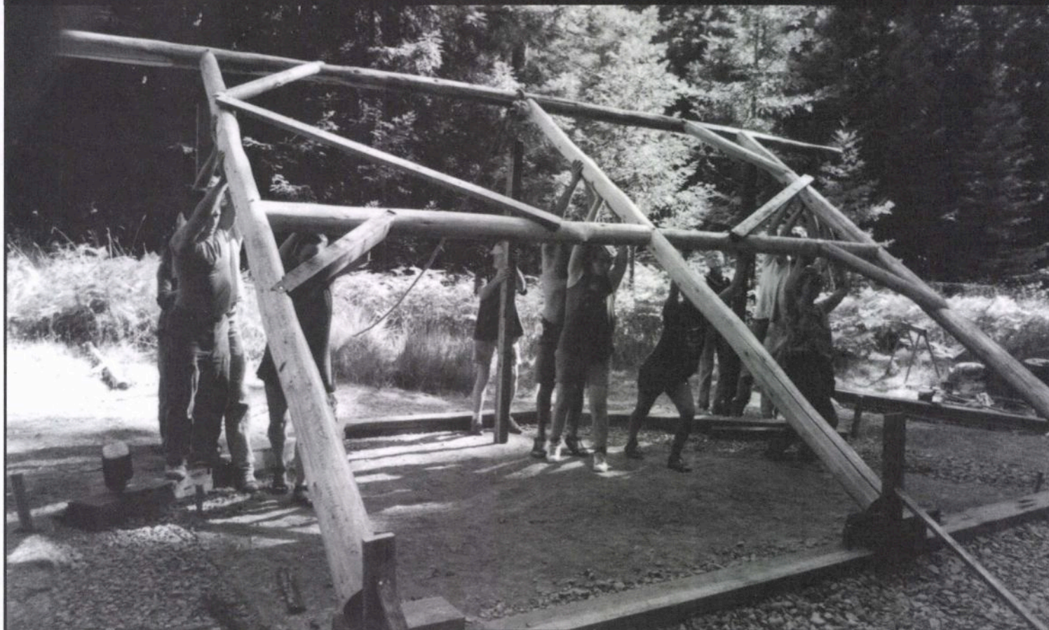
Raising a timber frame the old-fashioned way is the quintessential work party experience.
