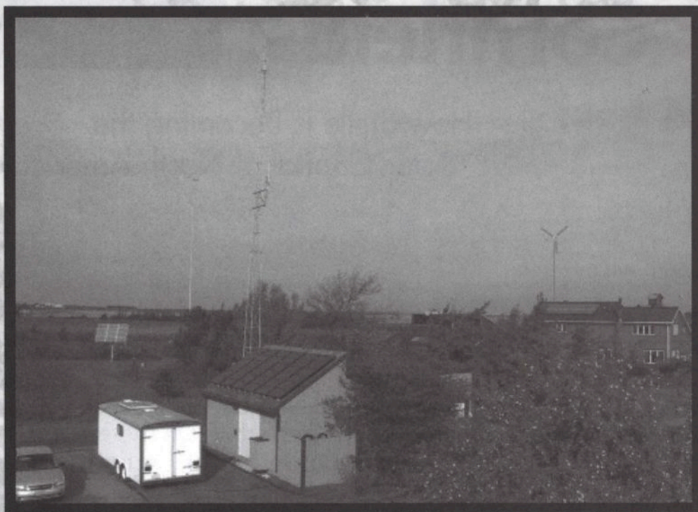
Stelle Phone Company generates power from PV panels on the roof; the solar tracker adds more power for its Internet service. The wind generator helps power a home.
