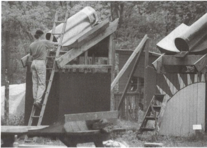
The Farm developed these parabolic collectors for solar hot water heating. At the Ecovillage Training Center (ETC), mid-1990s.
