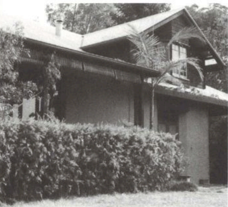
TOP: While the community uses grid power—conservatively—their new Education Centre and GEN office are solar powered.
