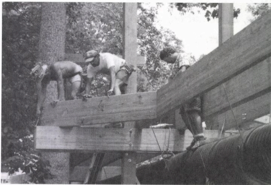
Erecting the pedestrian bridge between the two housing clusters. June, 1998.
