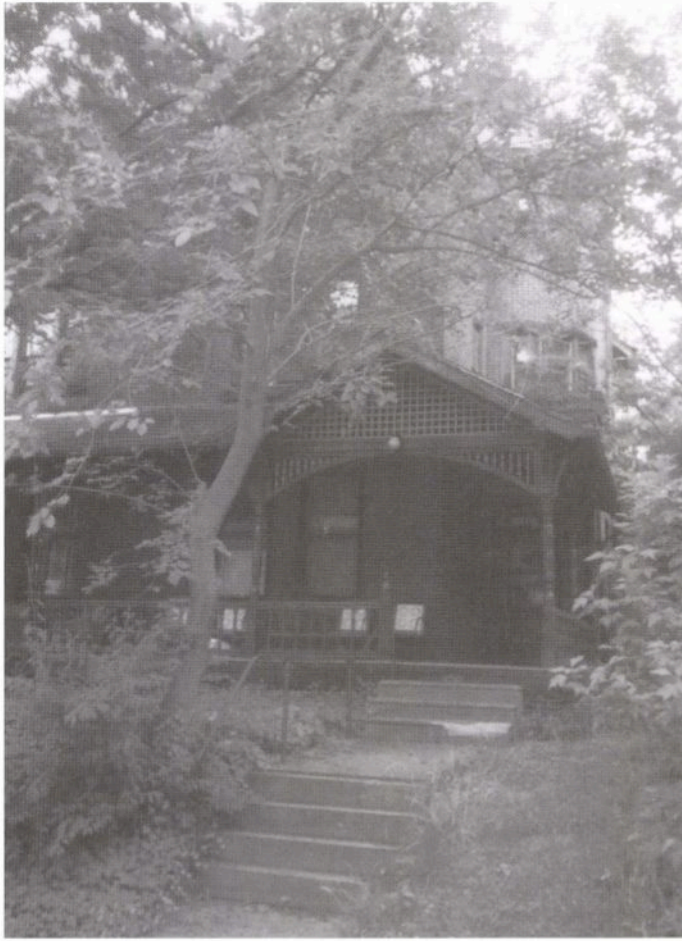
Oakshade, a small cooperative household, shares this Victorian home on a tree-lined street in West Philadelphia.
