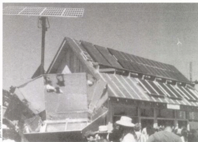
A large commercial (or community-sized!) solar oven being demonstrated in front of the MREA Demonstration Model Home. The home is built at the site of the annual fair at the fairgrounds in Amherst, Wisconsin, and shows off the best of renewable energy equipment.
